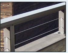
Corrosion damage created by electrolysis has occurred, due to the reaction between the stainless steel cables, the aluminum posts, and exposure to salt in the air.
