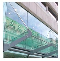
Designed to support loads in both tension and compression conditions, the rod assemblies can be used in a variety of structural and decorative applications – from glass curtain walls and door canopy supports, to guardrail balusters, to overhead awnings and trellis infill grids.
